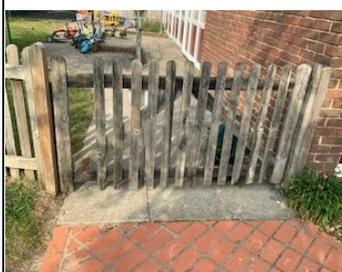
Even though we have attempted to repair this gate, it is just too heavy and continues to drop. Can you re-build it as a main master gate and smaller slave gate if we need full access?
