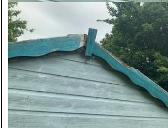
Re-felt the roof and replace the batten and fascias.
