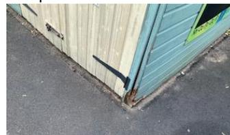
Replace the rotten side batten and it also needs a lick of paint!
