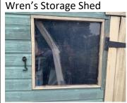
Replace the broken window with Perspex
