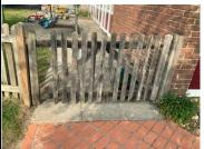
Even though we have attempted to repair this gate, it is just too heavy and continues to drop. Can you re-build it as a main master gate and smaller slave gate if we need full access?
