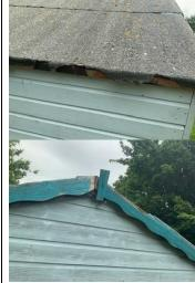
Re-felt the roof and replace the battens and fascias.
